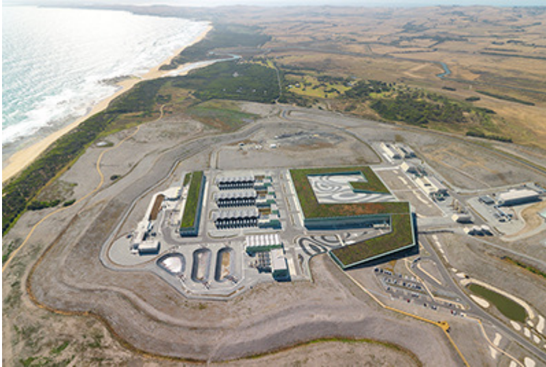
Caption: The VDP has a production capacity of up to 150 billion litres of water a year
