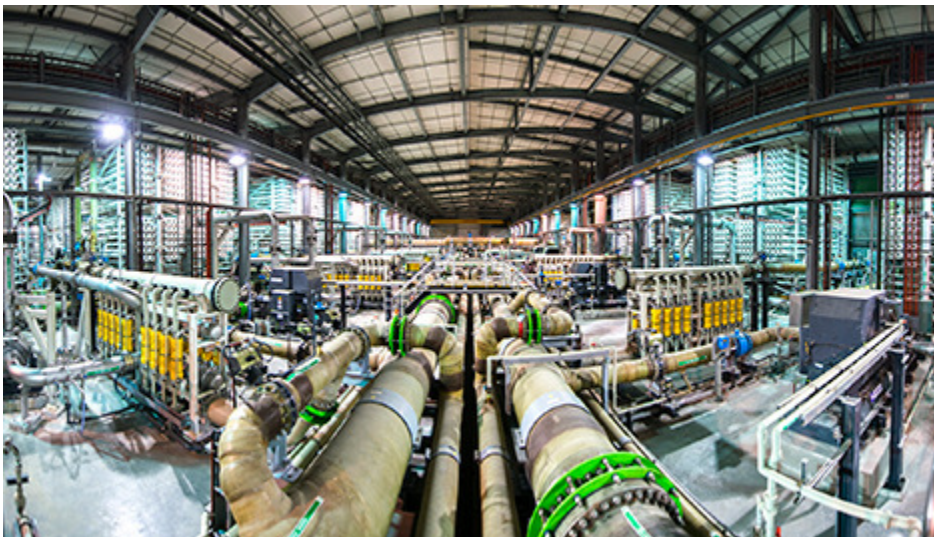
Caption: One of the main requirements for compressed air on the VDP is to actuate a number of the 17,000 plus automated valves
