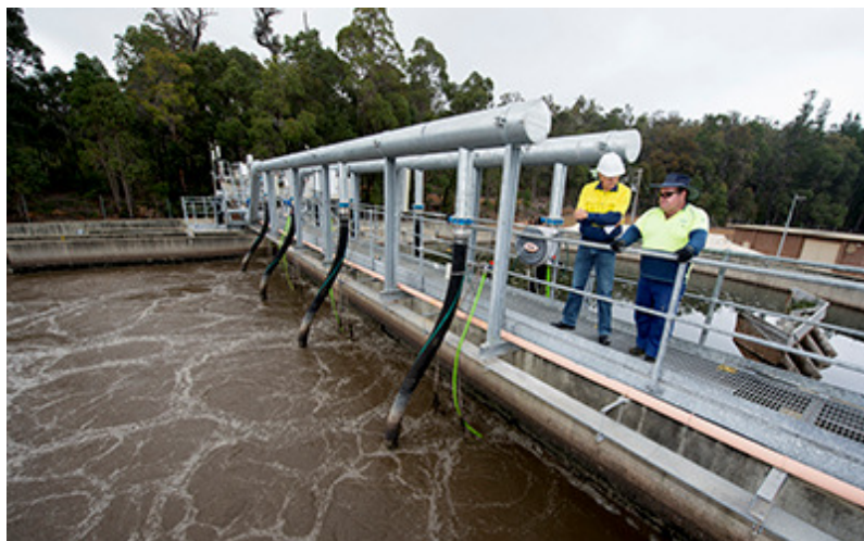
Caption: From aeration to digestion, a reliable and high quality supply of compressed air is required
