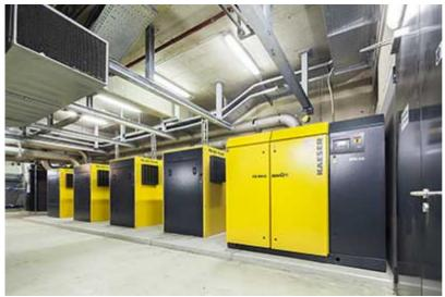
A clever component layout ensures that these units can easily be installed directly next to a wall, or side-by-side, additionally making maintenance easy.
