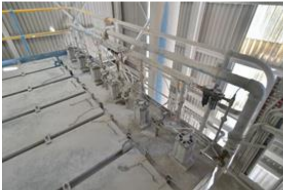
Caption: Compressed air is an essential utility required throughout the cement manufacturing process, from facilitating the flow of materials from start to finish, to assisting with the actual manufacturing process itself. Pictured above some dust collectors.
