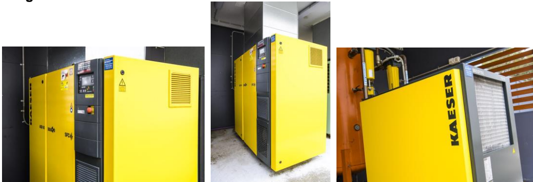
Caption for above selection of photos: The Kaeser ASD 60 SFC rotary screw compressor with Sigma Frequency Control complete with an air treatment package at Master Benchtops.
