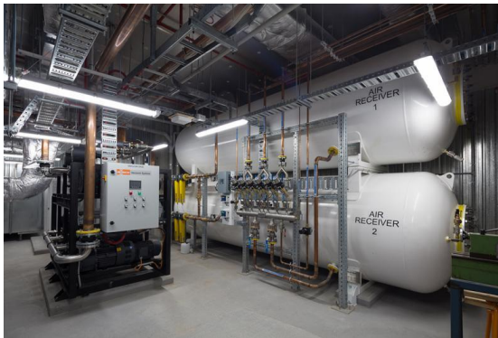
Caption: The compressed air treatment package includes Kaeser filters - the key component to produce compressed air to all purity classes as per ISO 8573-1.
