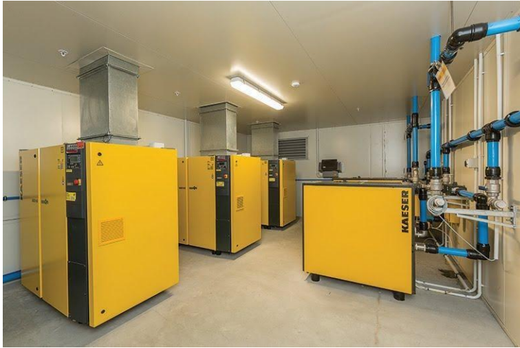
Caption: The complete Kaeser compressed air system that was recently installed at Tasti Foods.
