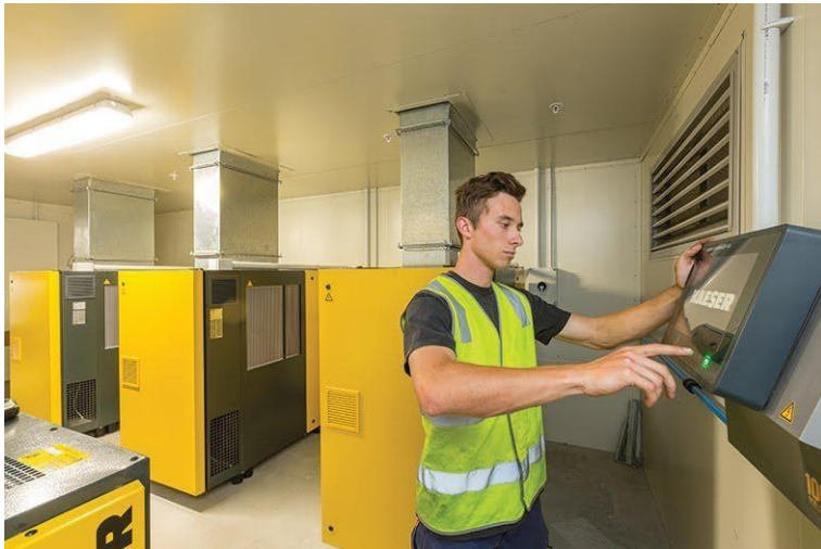
Caption: For maximum efficiency, complete control and connectivity of all components within the compressed air station, a SAM 4.0 master controller was installed.
