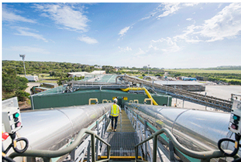
Caption: The biosolids storage and outloading facility at Malabar WWTP
