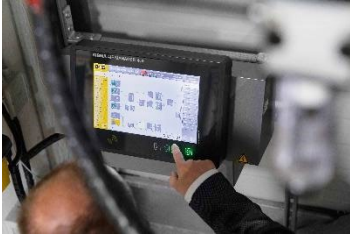
Caption: Compressed air management systems such as the Sigma Air Manager 4.0 are the centrepiece of a modern air station.
