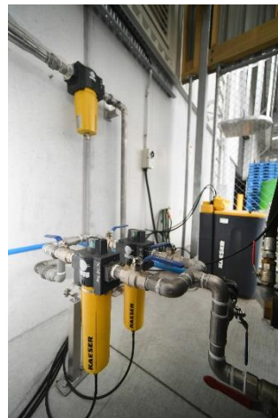
Caption: The Kaeser Aircenter all-in-one compressed air station, complete with filtration at Suntory Coffee.
