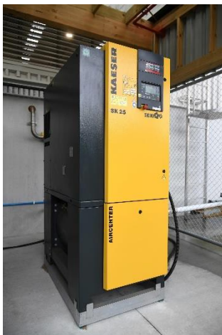
Caption: The Kaeser Aircenter all-in-one compressed air station, complete with filtration at Suntory Coffee.
